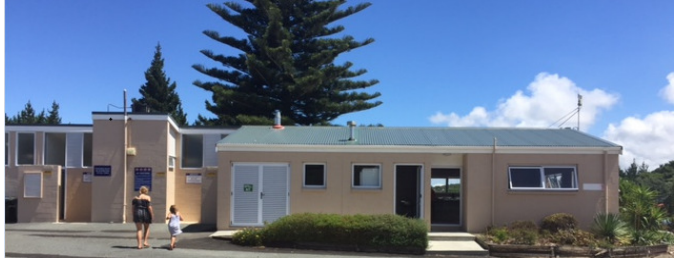
Crem Block Kitchen Extension $128,056
